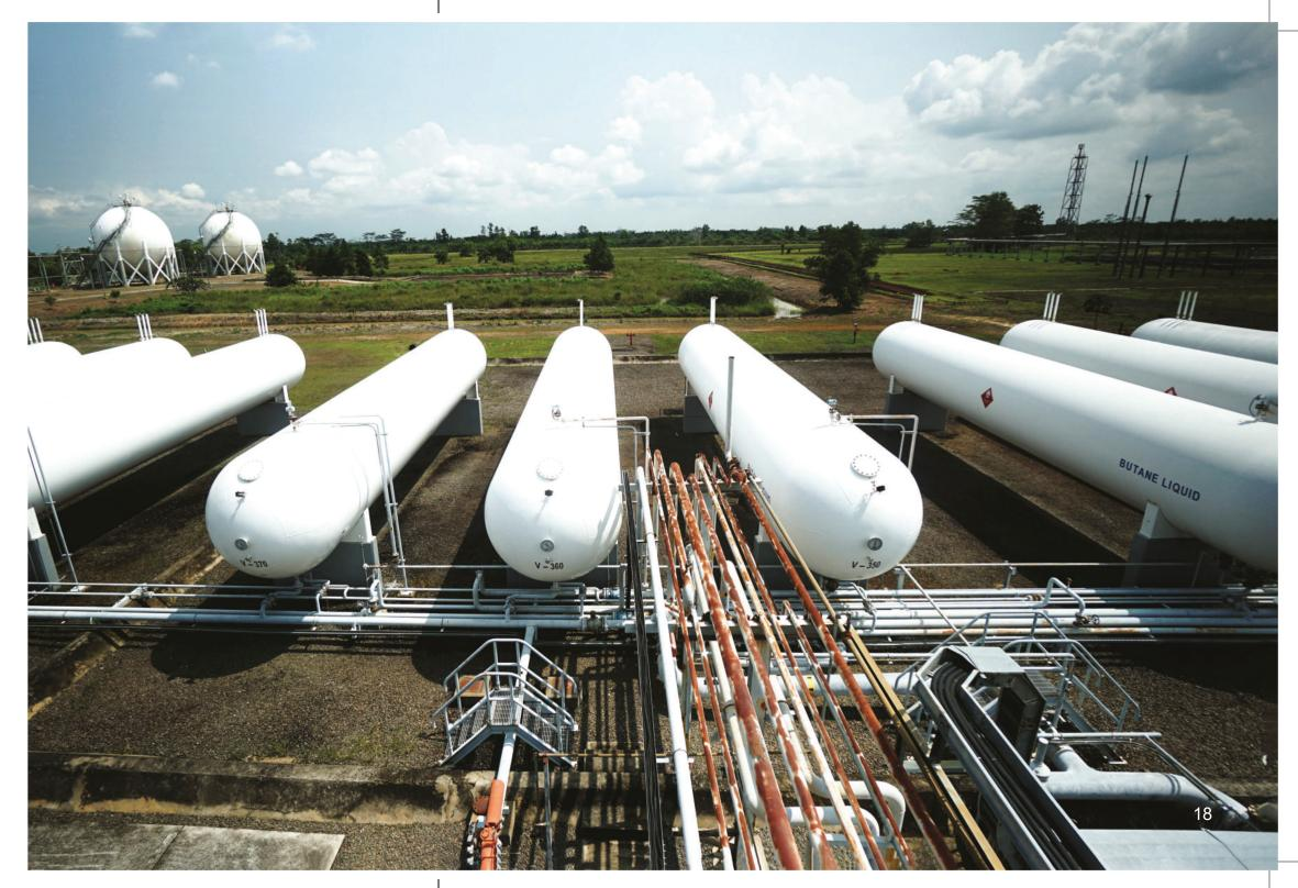
The North Geragai Fractionation, which processes the low CO2 gas and natural gas liquid from Betara Gas Plant, as well as PetroChina's oil fields around Geragai. The facility separates propane, butane, ethane and condensate before being transferred to Fixed Processing Unit.
