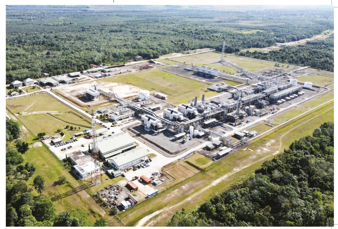
In Betara Gas Plant, we process the high CO2 gas from PetroChina's oil fields in Betara area. Operated in 2005, BGP separates methane and ethane and has the capacity of 241 MMSCFD (with 38-40 percent CO2 content).
